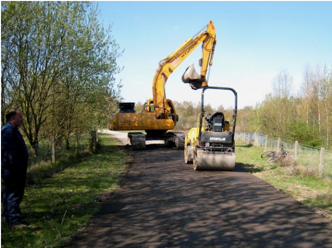
Path being laid through Walton Country Park earlier this year
