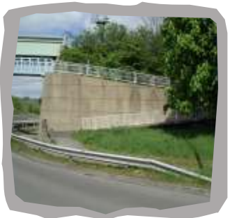
Footbridge over dual carriageway towards Sowgate Lane (Waymarker 11)
