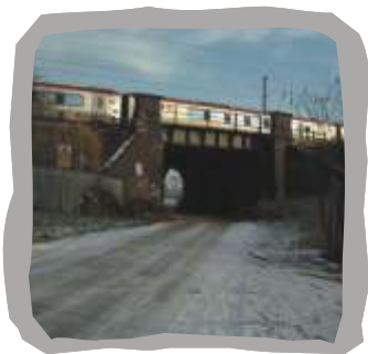
Railway bridge (Waymarker 1)
